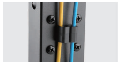
Cable management maintains a clean look.
